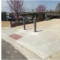
Curb Cut ADA Ramp with Bollards Image Credit: thewashcycle.com
