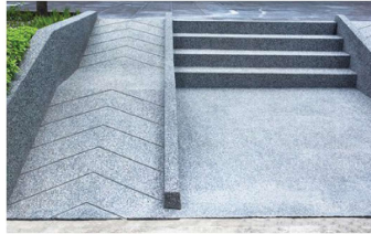
ADA Ramp with Adjacent Stairs [Note: All Ramps and Stairs to Include Railing] Image Credit: 123RF.com
