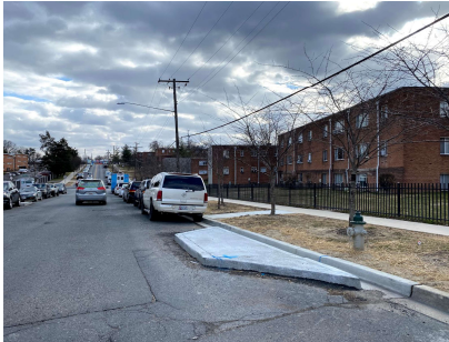
Mid-Block Curb Extension
