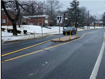
Concrete Spot Median Island
