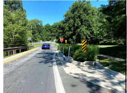
Stormwater Swale in Curb Extension
